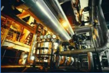
CUNO Filtration Systems For Automotive Assembly Plant
